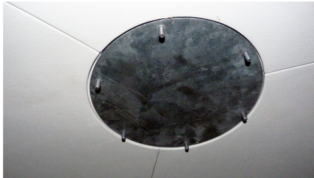
Photo of center plate bolted to center hub. The center hub sits on the back of the dish. Bolted together these two pieces 'pinch' the reflector and are part of the main support structure.
