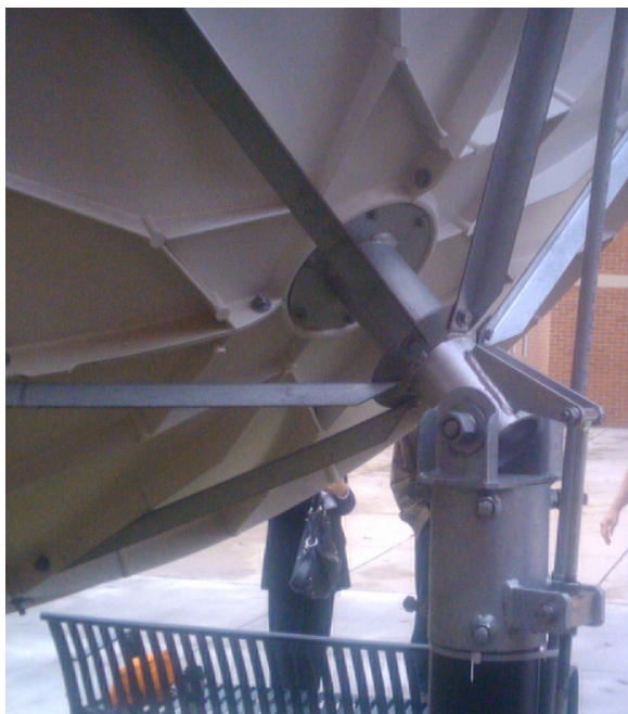
Back of the dish showing the support assembly attached to the canister and elevation assembly.
